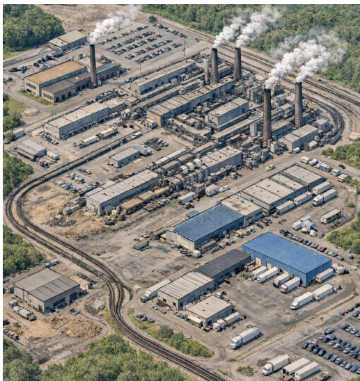
Drone photograph of Rodgers Paper Mill
